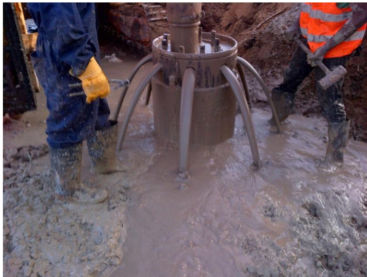
Picture of Concreting of Pile
