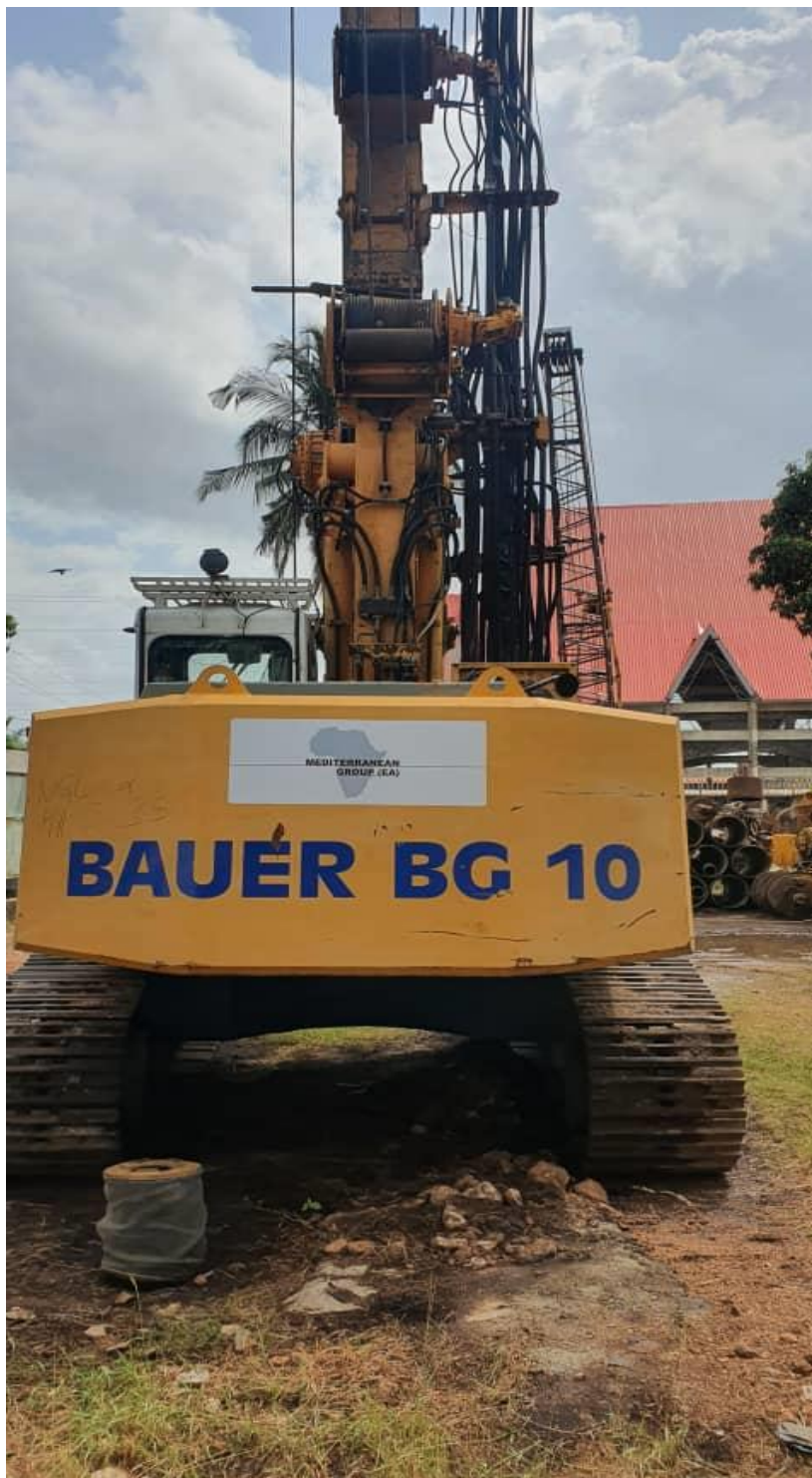
Bauer BG10, Drilling Rig
