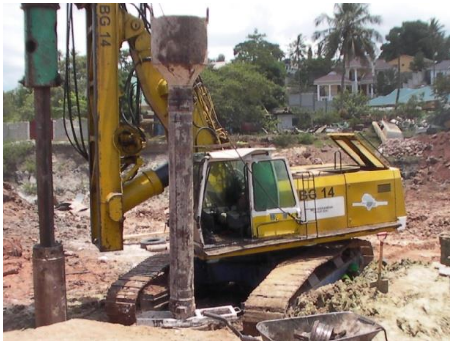
BG 14 Big Diameter Drilling Rig for Kinyerezi Bridge Dar Es Salaam, Tanzania - ( 68 Piles diameter 600 mm )
