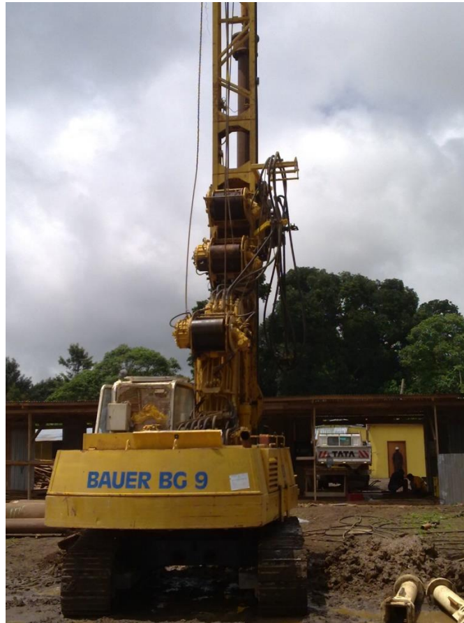
Bauer BG-9 Drilling Rig
