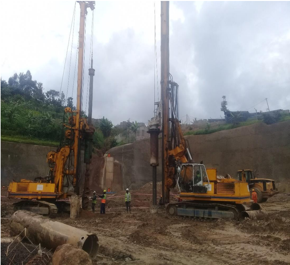
Foundation Works, Gas Plant, Rwanda
