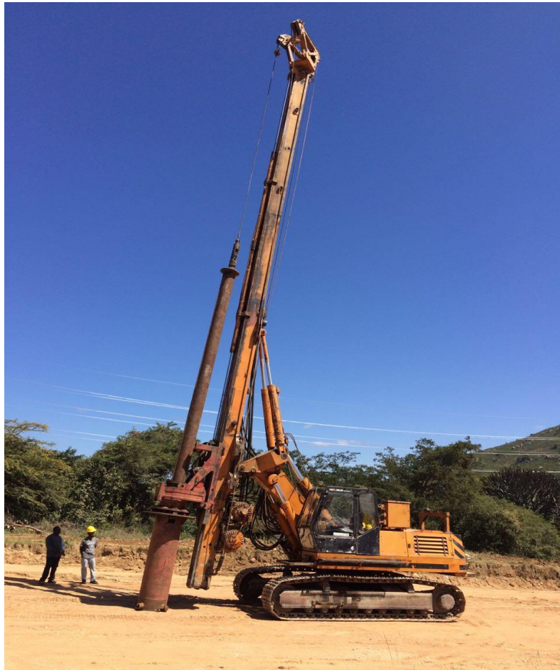
Delmag RH 0912 Drilling Rig
