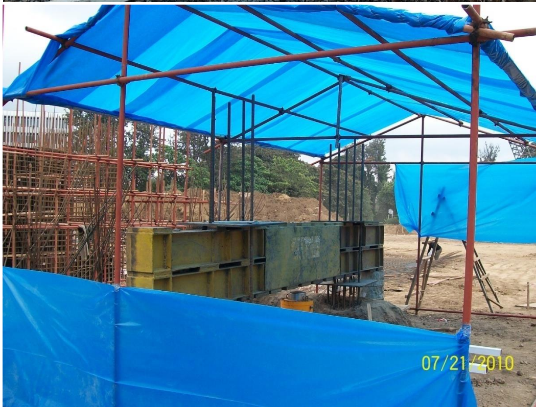
Pile Load Testing
