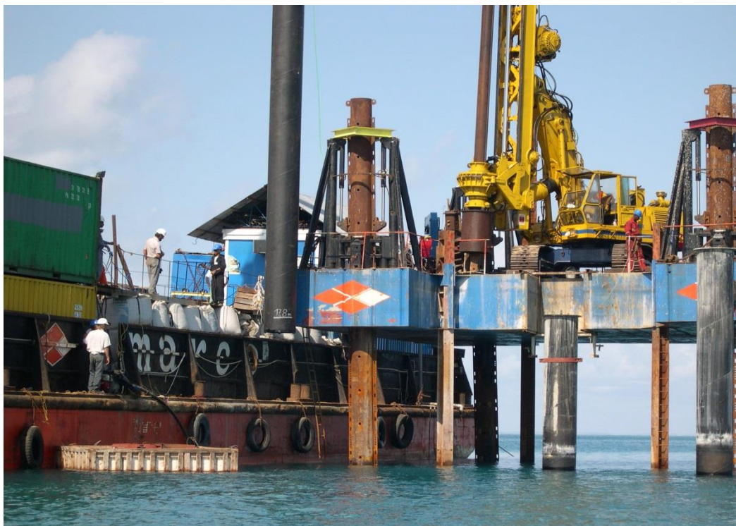
Big Diameter BG 11 Drilling Rig on Jack Up Pontoon (76 Piles diam. 1000 mm for Offshore Foundation Works Songo Songo, Tanzania )
