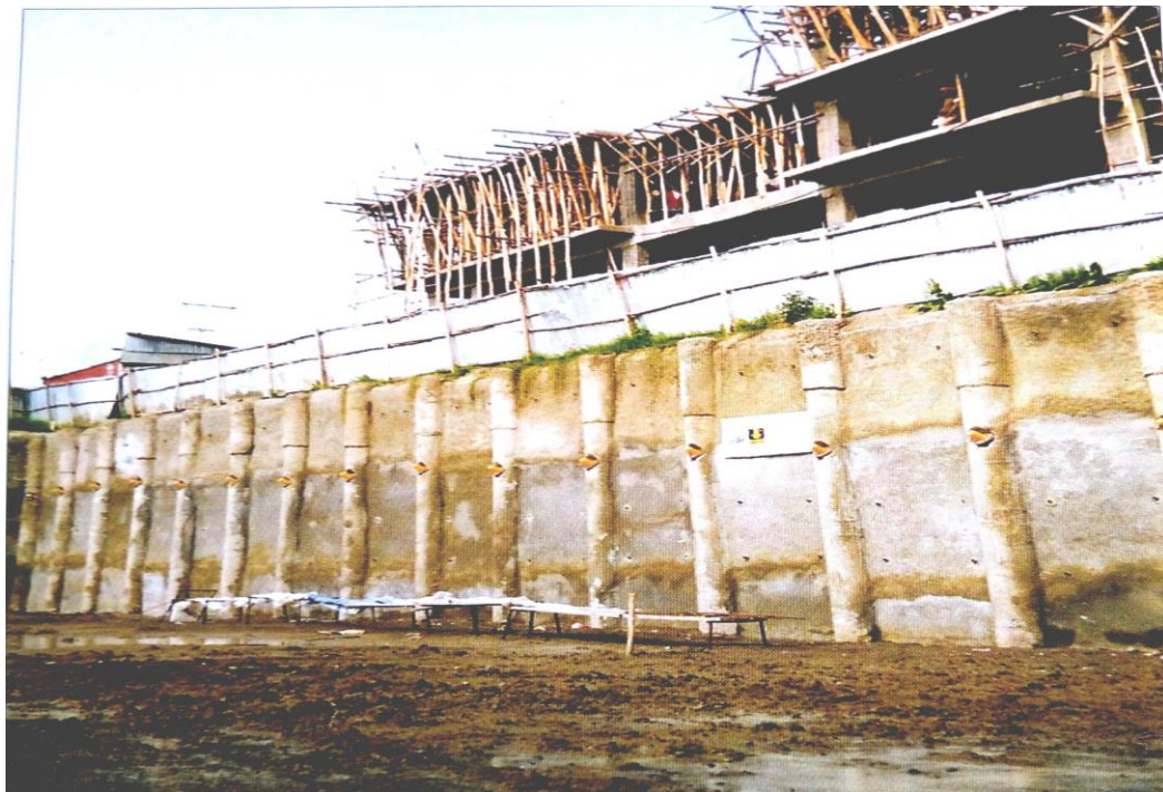
Inner City Shoring Works for 3 story Underground Parking- Addis Ababa
