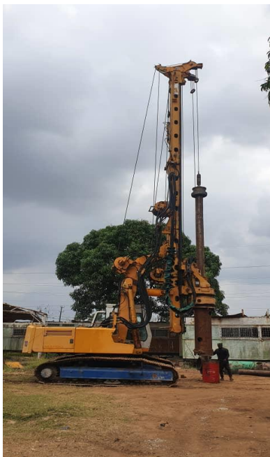
Bauer BG 10 Drilling Rig
