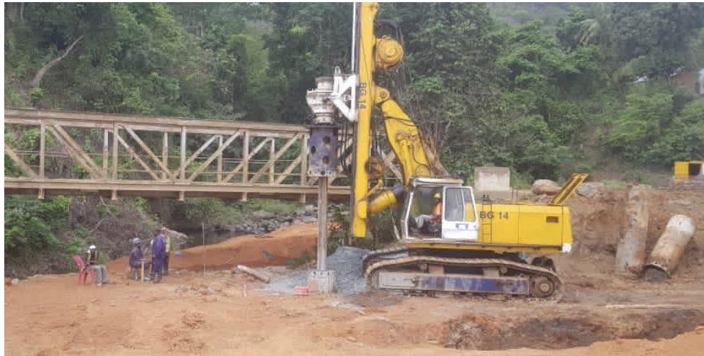
Pile Drilling in a River Bed
