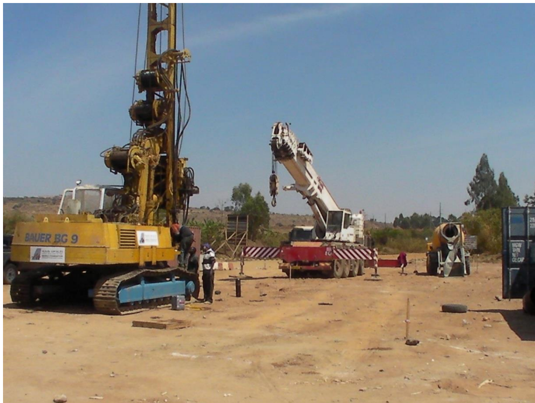
BG 9 Big Diameter Drilling Rig ( 109 Piles diam. 600 mm in Sumbawanga Leila Bridge, Tanzania)
