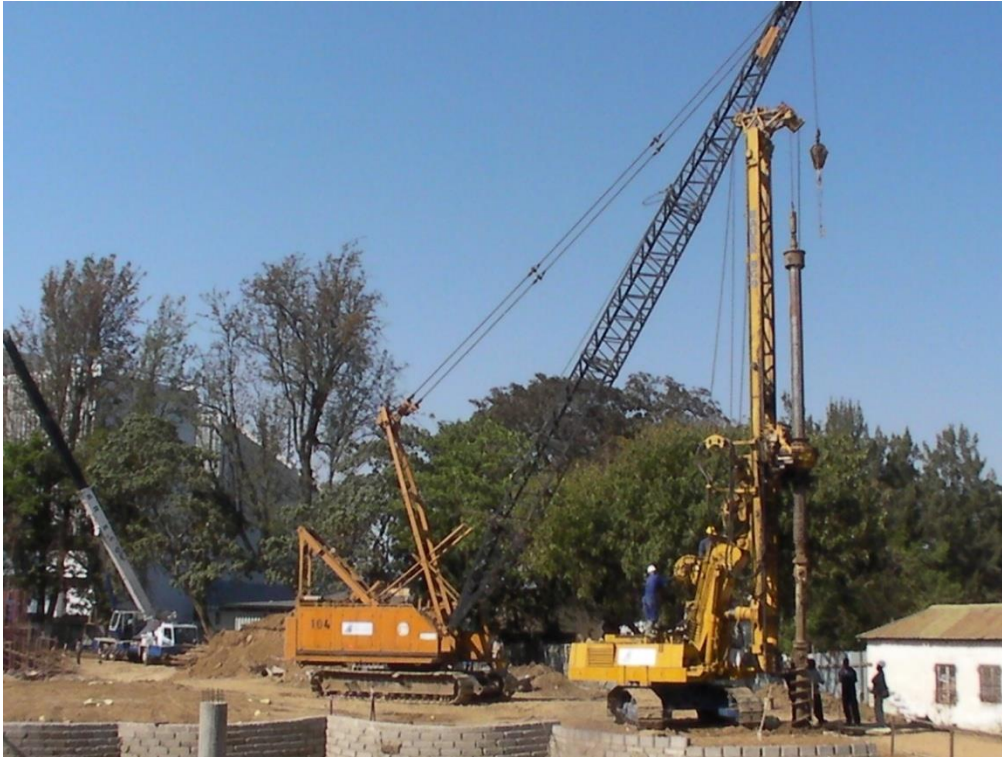
65 ton Crawler Crane and BG 9 Drilling Rig ( EAC Head Office in Arusha 262 Piles diam. 620 mm , 262 Integrity Test, 3 Load Tests )
