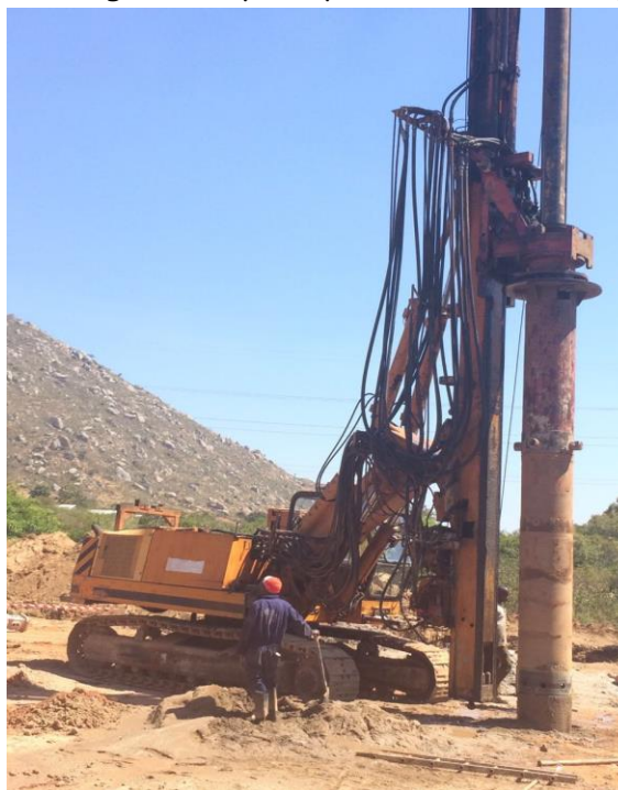
Placing of Temporary Douoble Wall Casing
