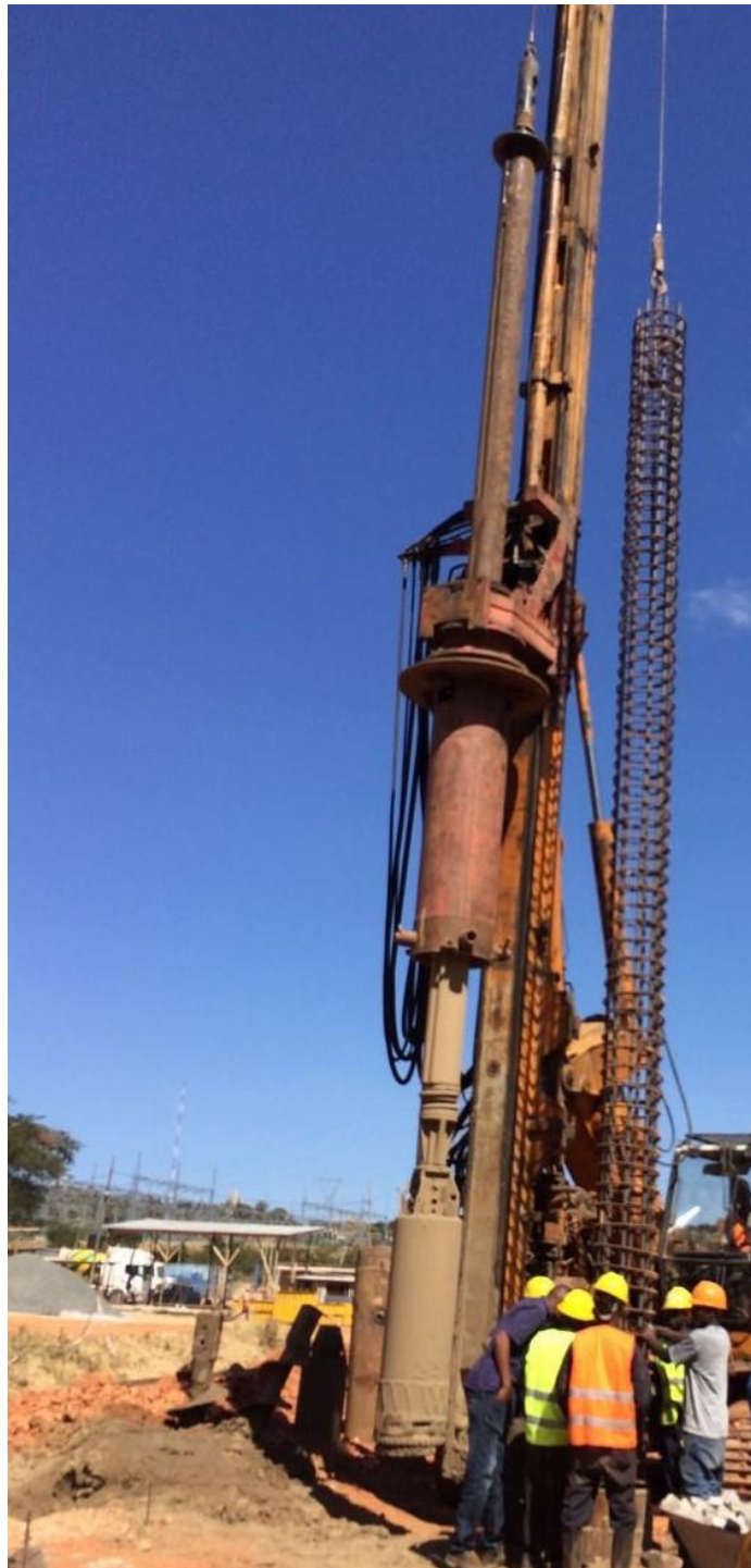
Installation of Reinforcement Cage
