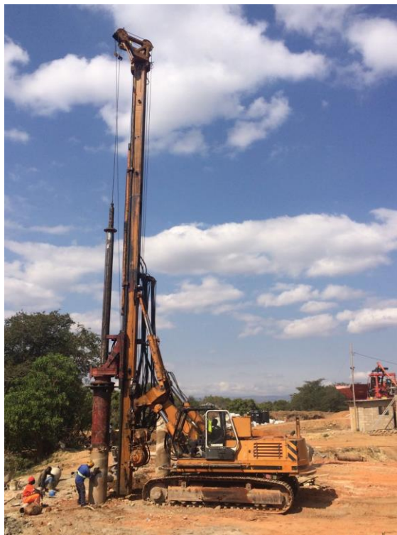
Placing of Temporary Double Wall Casing
