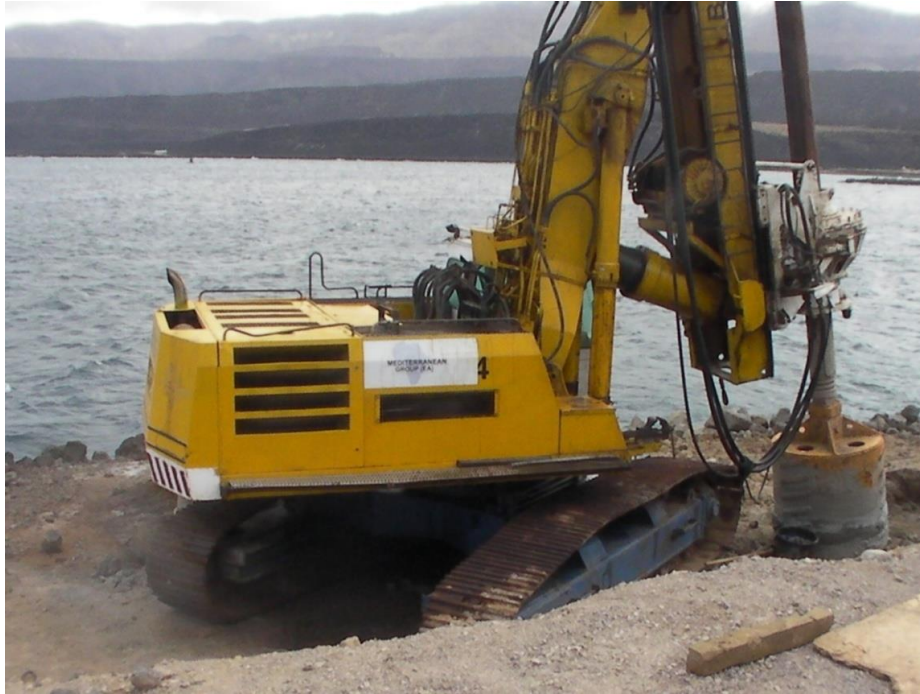
BG 14 Big Diameter Drilling Rig for Salt Exportation Port in Djibouti - ( 98 Off Shore Piles diameter 1200 mm drilled from barge, 9 Piles on Shore)
