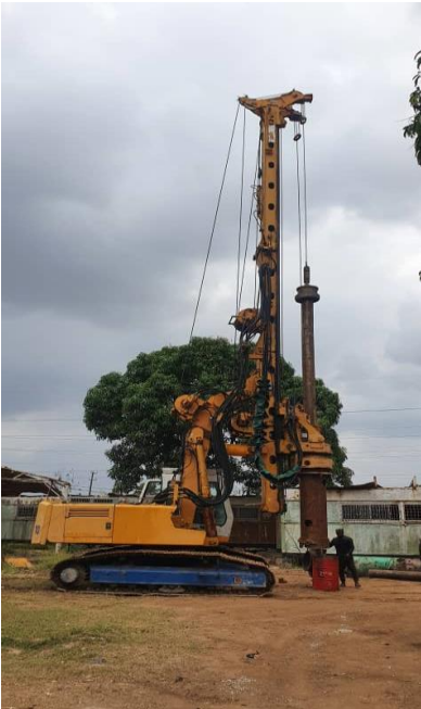
Bauer BG 10 Drilling Rig
