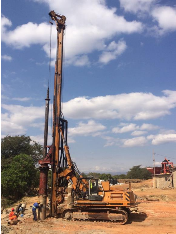
Placing of Temporary Double Wall Casing
