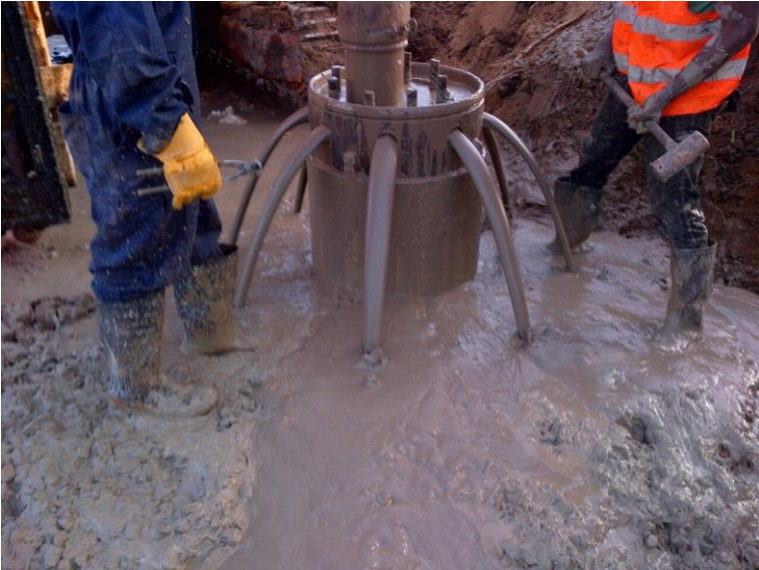
Picture of Concreting of Pile
