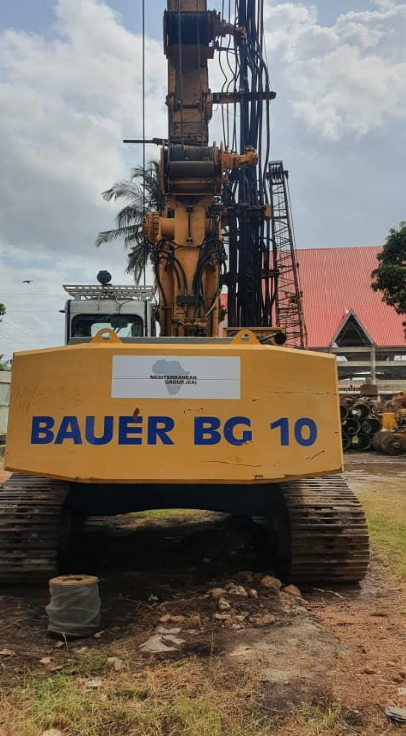
Bauer BG10, Drilling Rig
