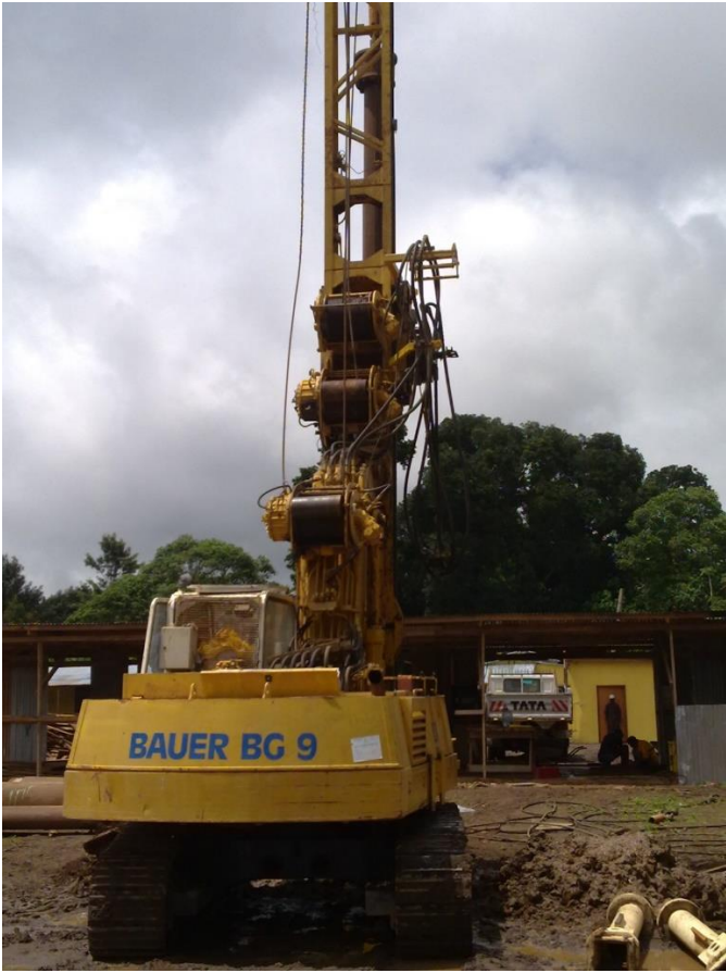
Bauer BG-9 Drilling Rig
