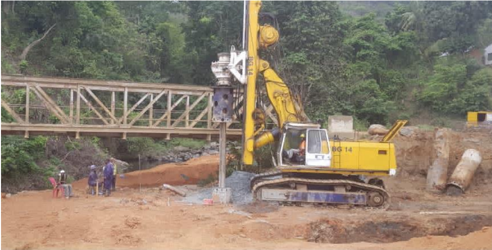
Pile Drilling in a River Bed
