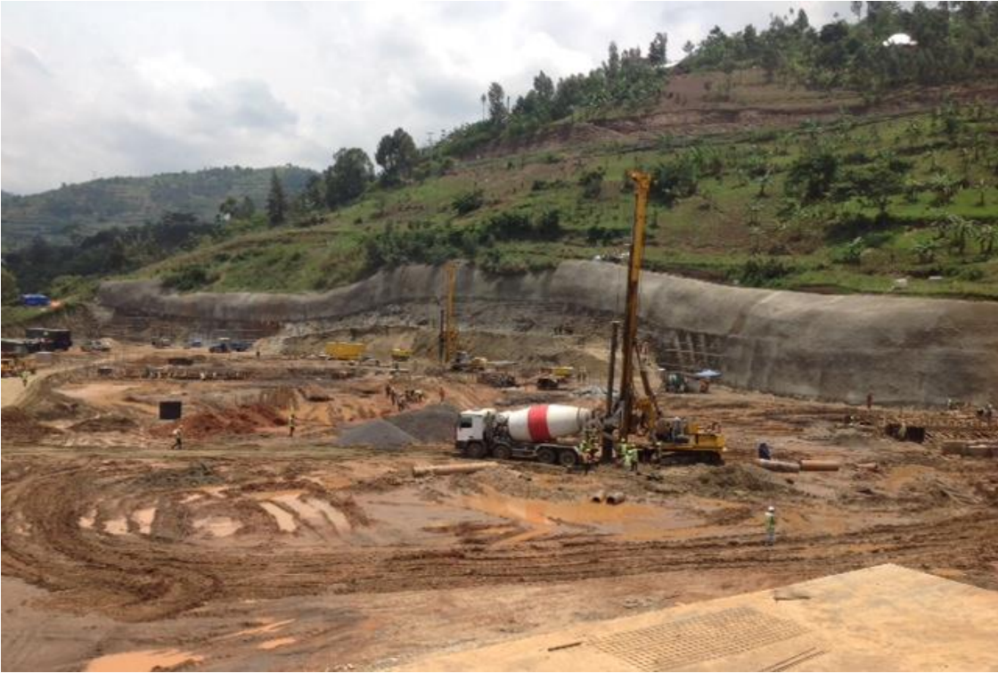
Foundation Works, K56 Gas Power Plant, Lake Kivu, Rwanda
