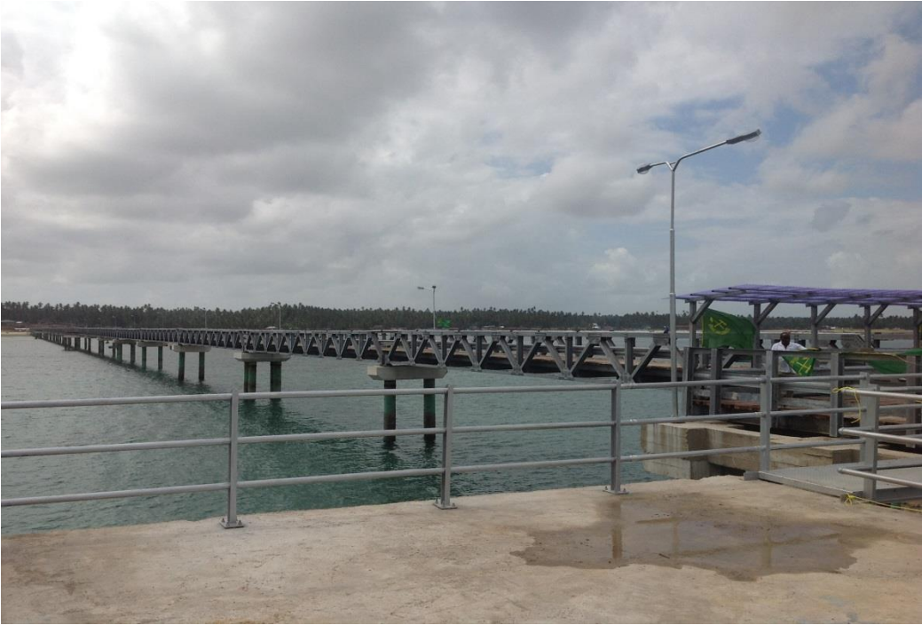
Offshore Bridge Project Mafia Island, Tanzania (109 Off Shore Piles diam. 800 mm)
