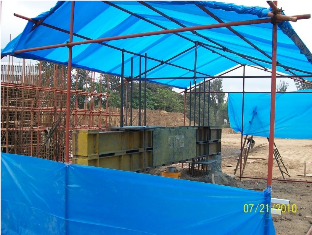
Pile Load Testing
