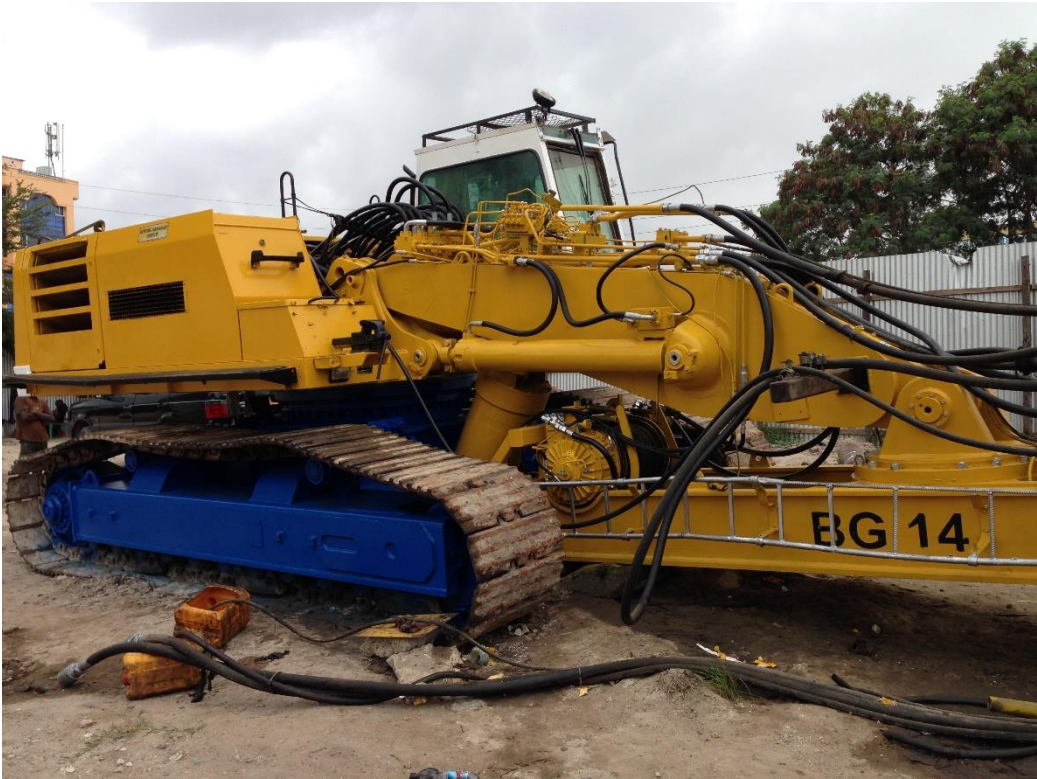
BAUER BG 14 Drilling Rig
