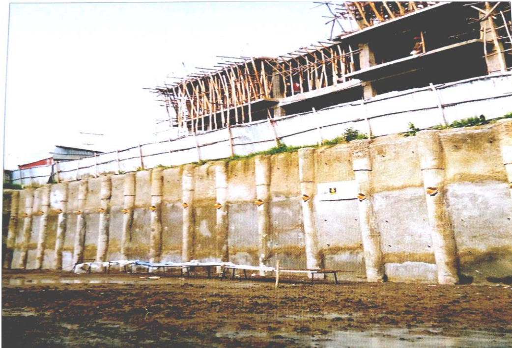
Foundation Project in Addis Ababa, Ethiopia (316 Piles diam. 880 mm)
