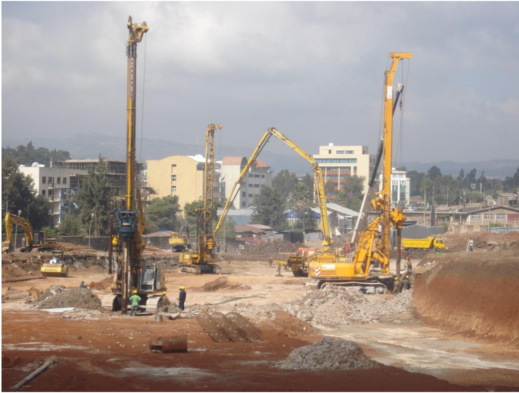
Foundation Project in Addis Ababa, Ethiopia (316 Piles diam. 880 mm)
