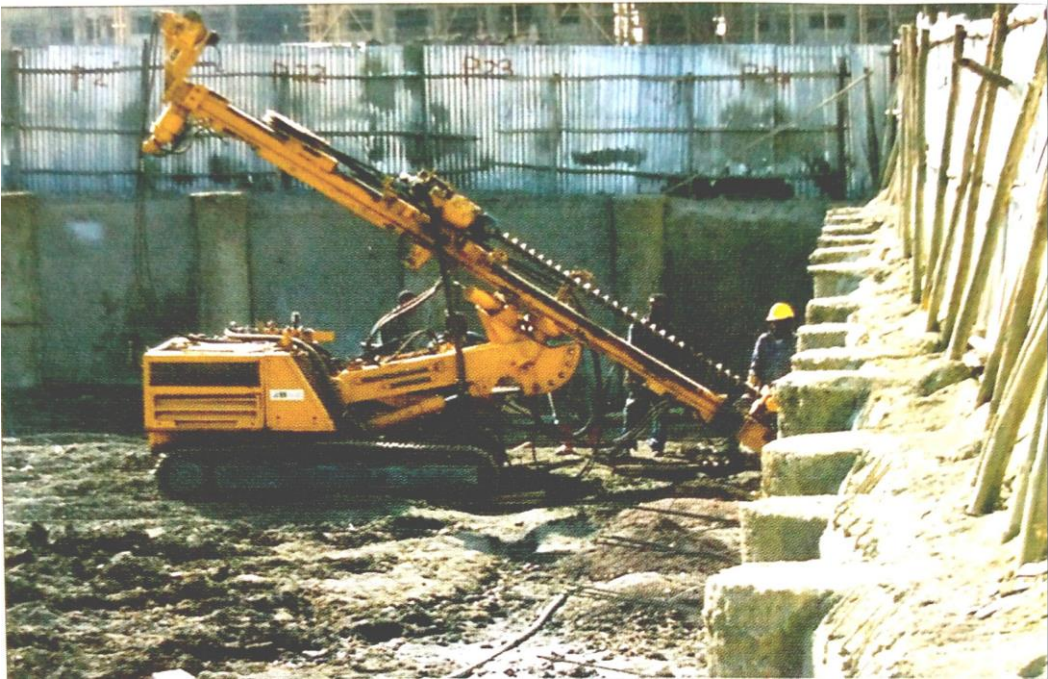
Grouted Anchors Installation for Shoring System- Addis Ababa
