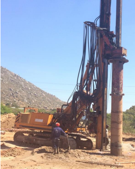
Placing of Temporary Double Wall Casing
