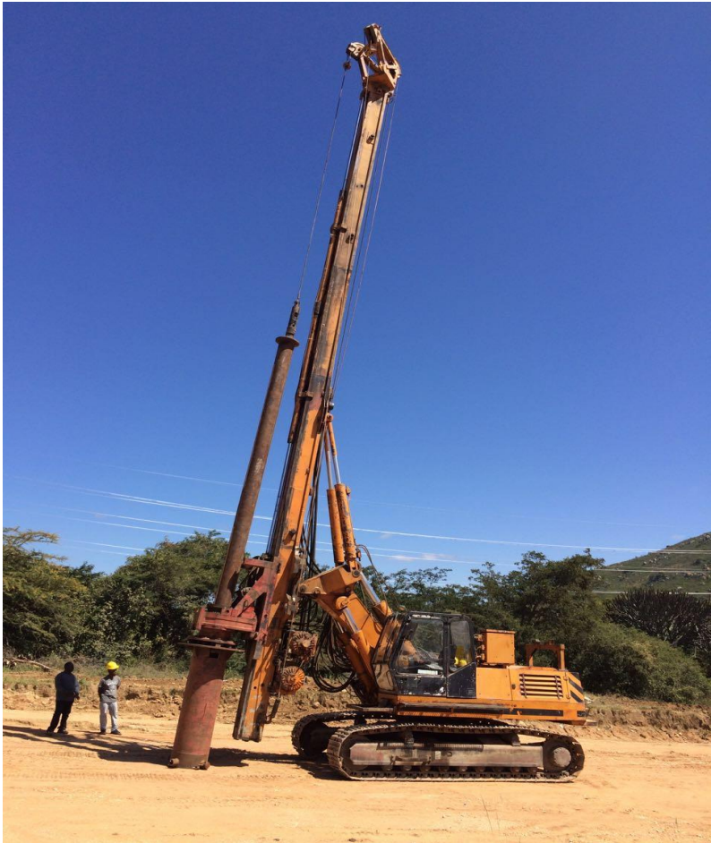
Delmag RH 0912 Drilling Rig
