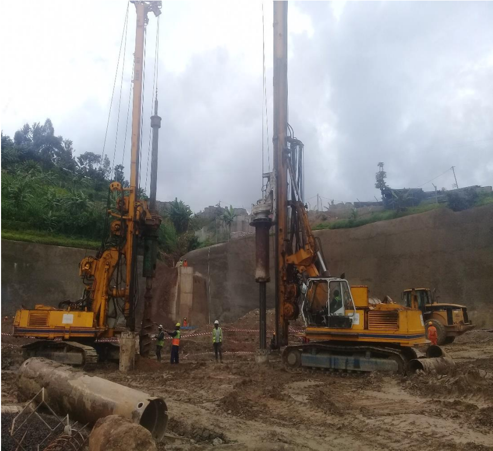
Foundation Works, Gas Plant, Rwanda
