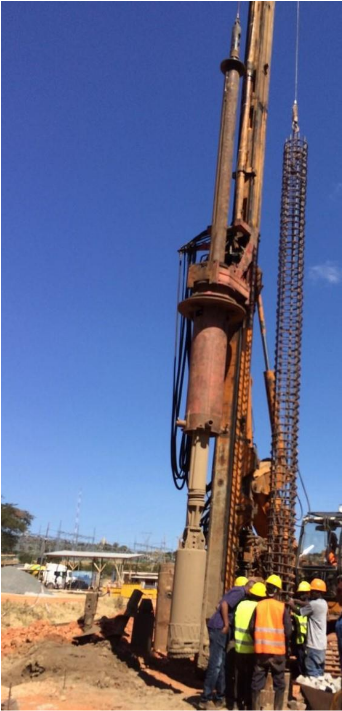
Installation of Reinforcement Cage
